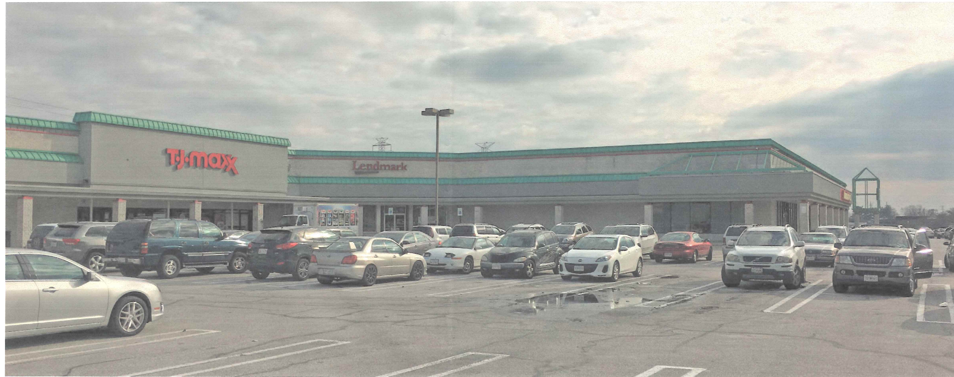
PHOTOGRAPHS OF ELEVATIONS A, B & C - BEFORE
