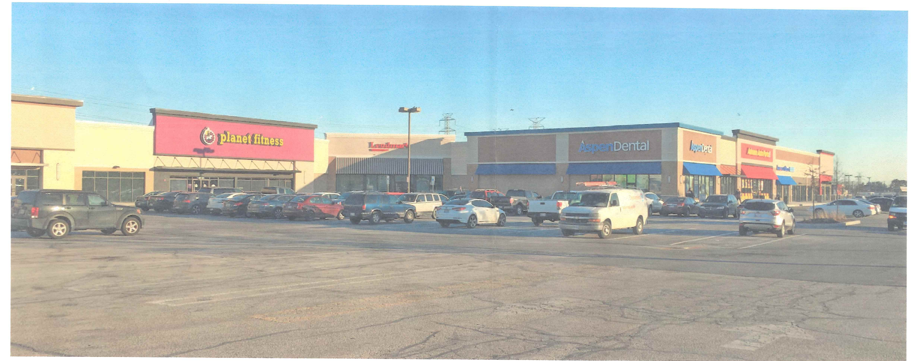
PHOTOGRAPHS OF ELEVATIONS A, B & C - AFTER
