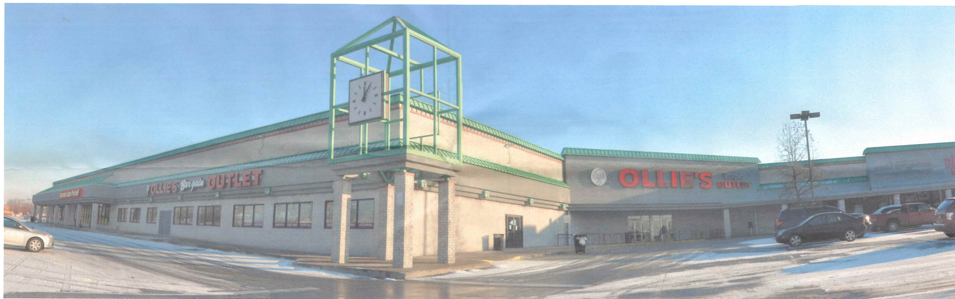
PHOTOGRAPHS OF ELEVATIONS, D, E, & F - BEFORE
