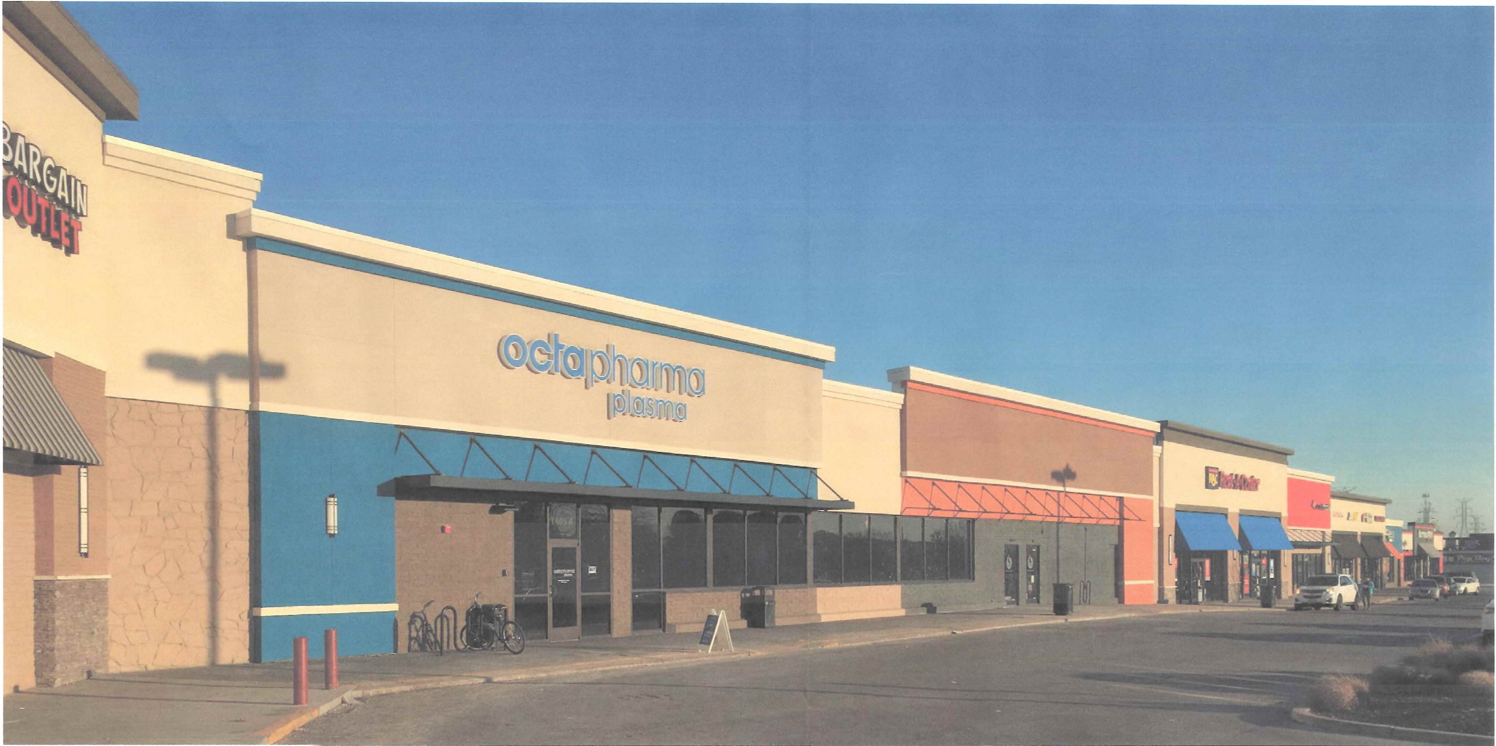
PHOTOGRAPH OF ELEVATION G LOOKING SOUTH - AFTER
