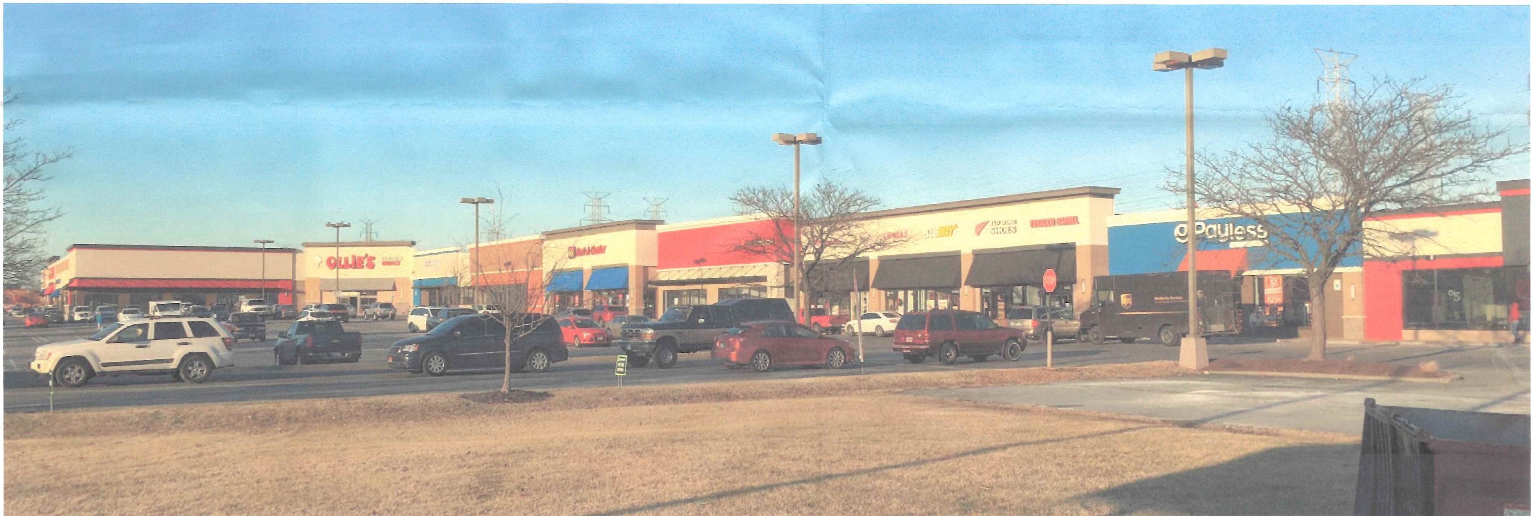
PHOTOGRAPH OF ELEVATIONS G & E LOOKING NORTH - AFTER
