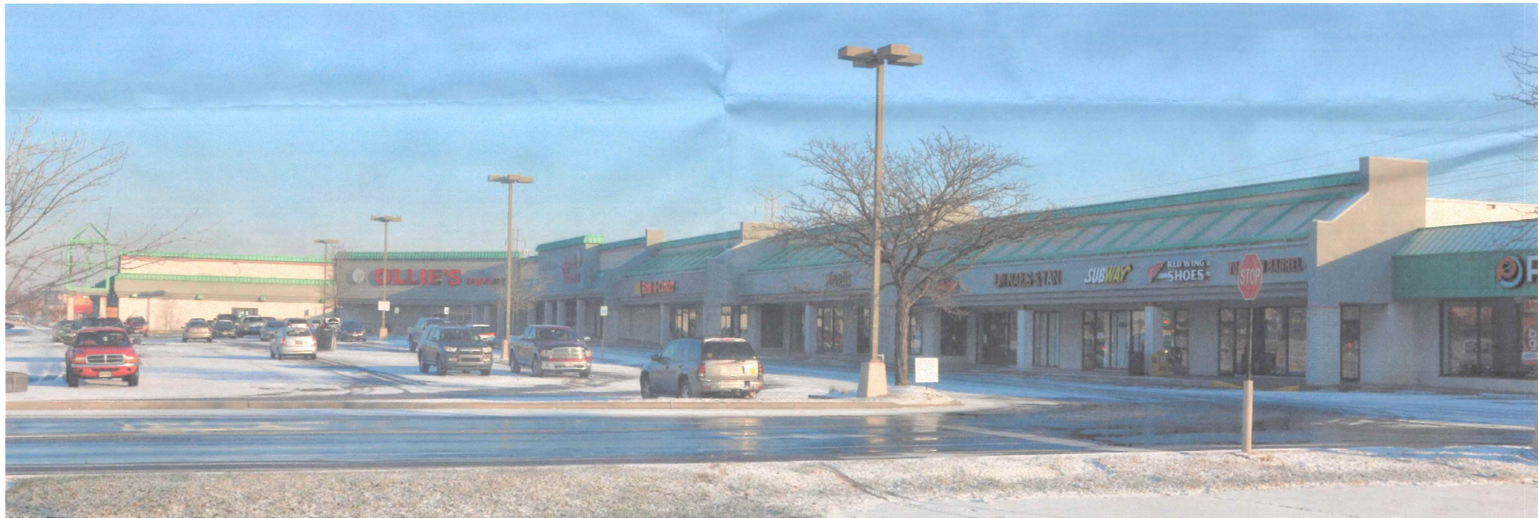
PHOTOGRAPH OF ELEVATIONS G & E LOOKING NORTH - BEFORE
