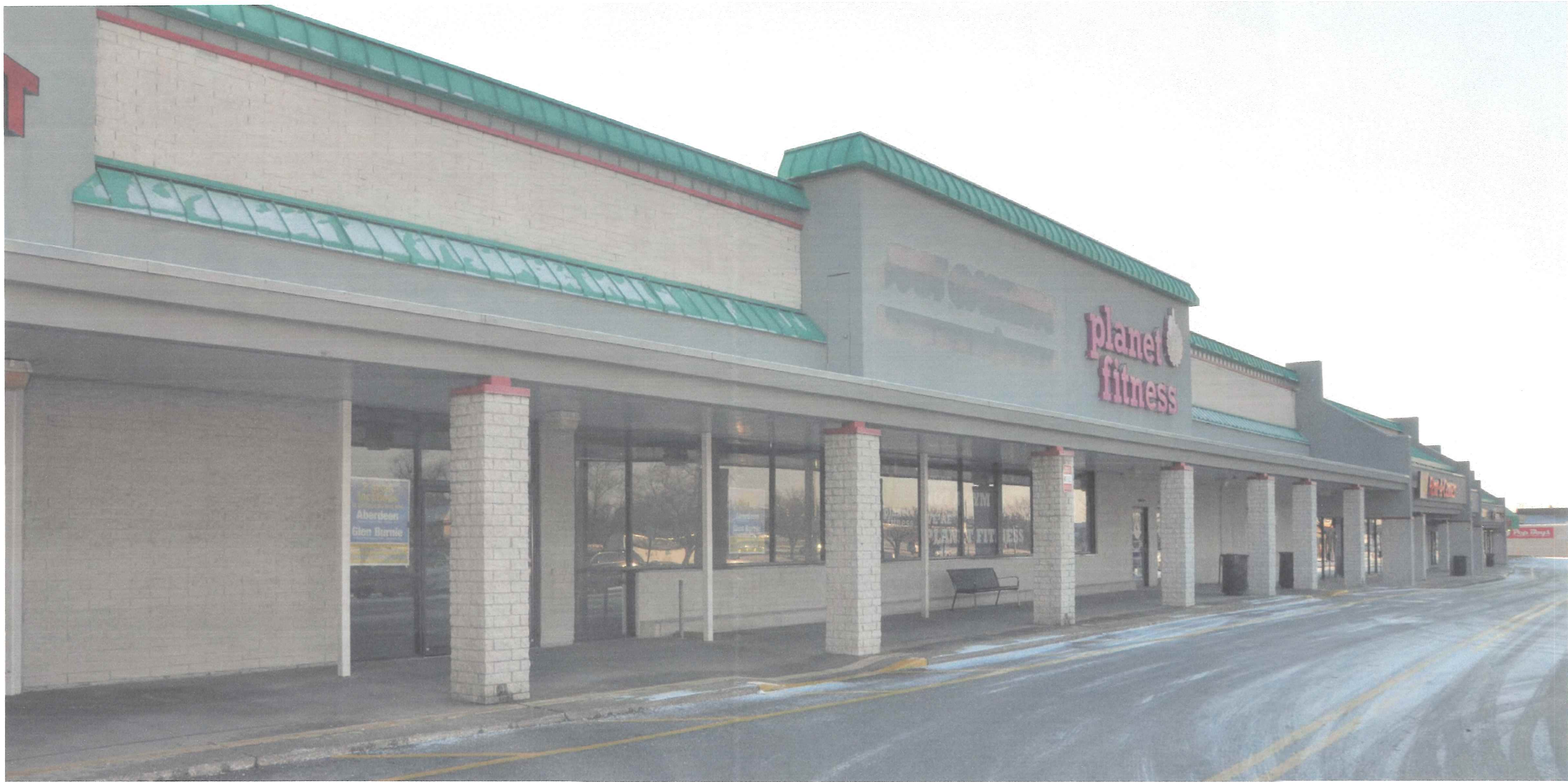
PHOTOGRAPH OF ELEVATION G LOOKING SOUTH - BEFORE
