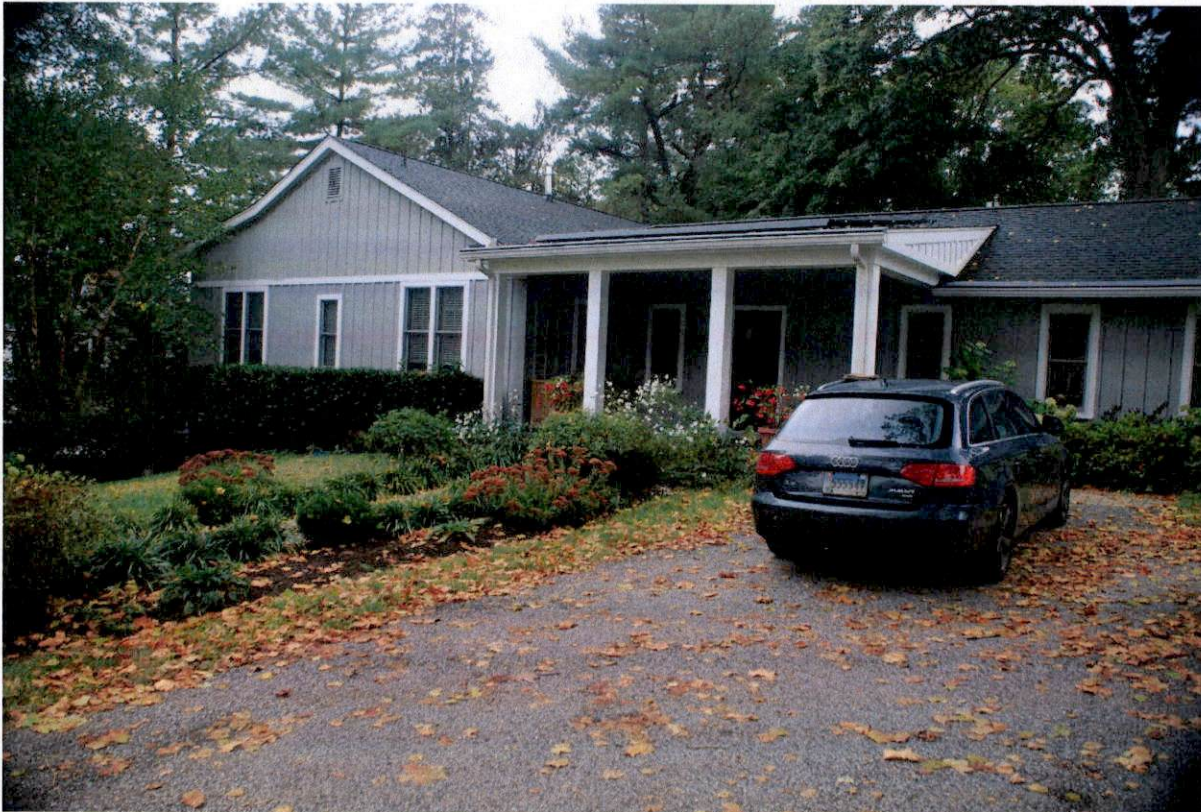
FRONT OF 7606 CURVING LANE - PROP. GARAGE RIGHT OF PORCH.
