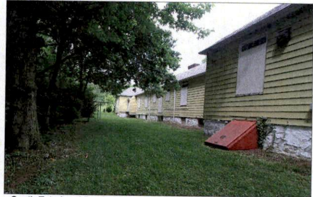
South Exterior - View West
