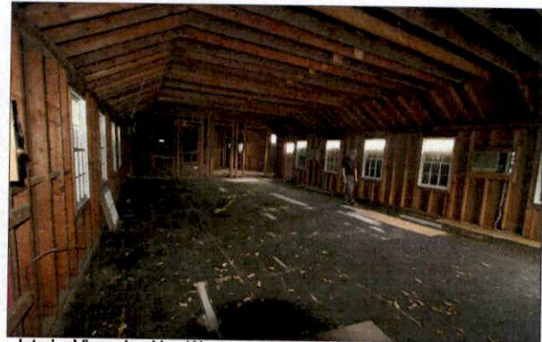
Interior View - Looking West
