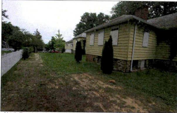
North Exterior - View East
