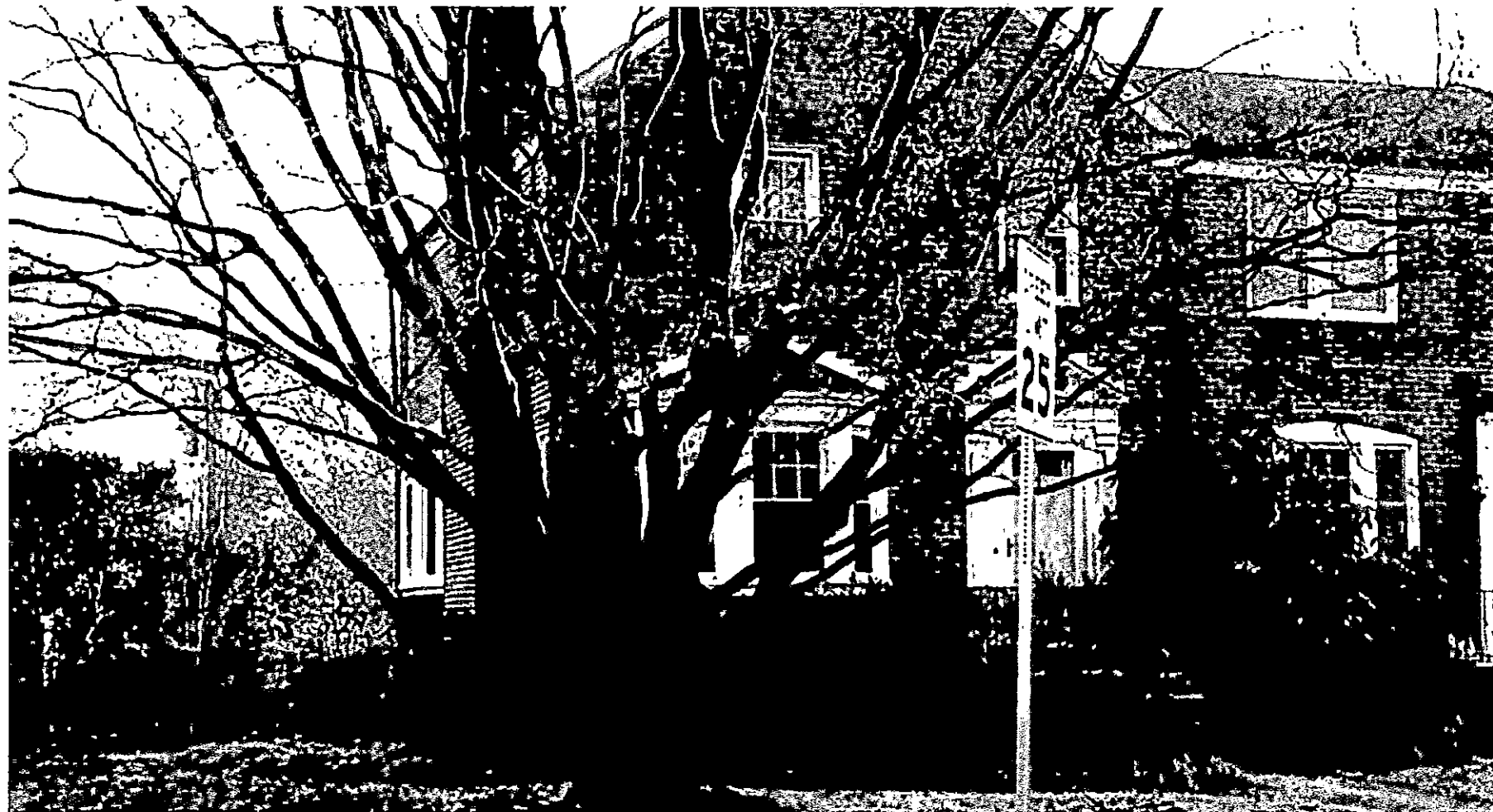
view of the front of 247 Blenheim
