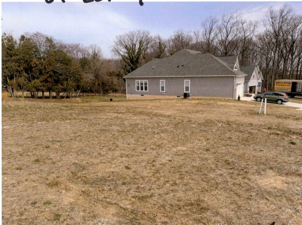
SIDE VIEW of House (Lot 4) NO House built on Lot 3 yet.
