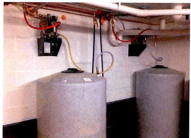
Basement Tank Room – steel and polypropylene tanks and secondary containment wall
