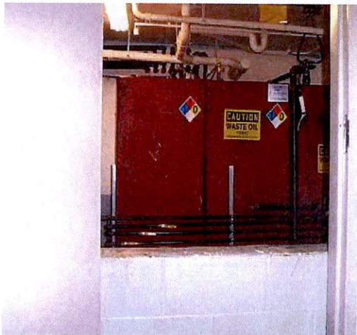
Basement Tank Room – steel and polypropylene tanks and secondary containment wall
