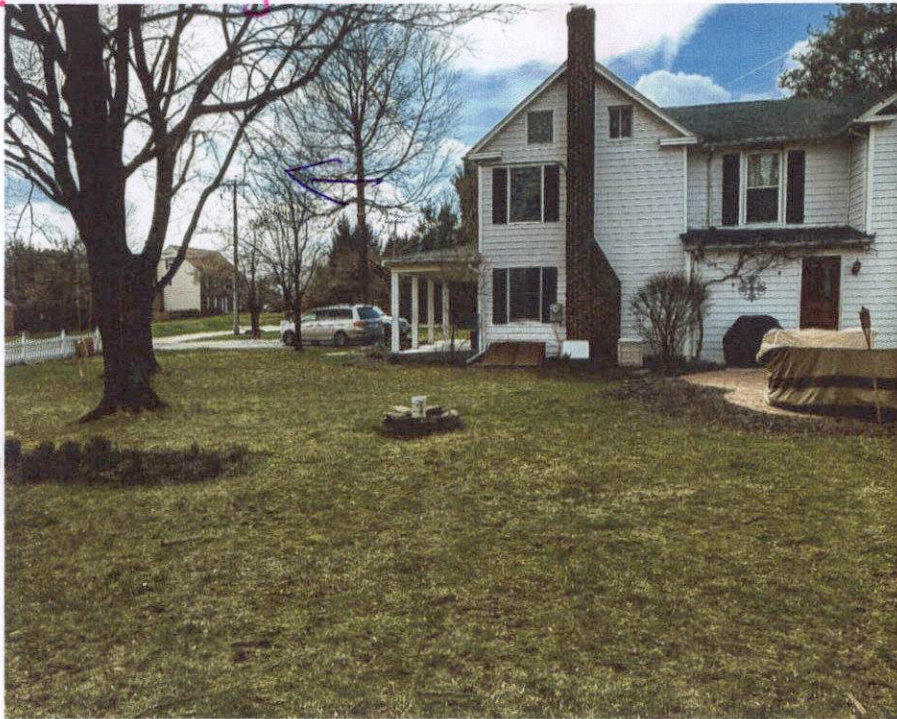
B. Photo facing west
