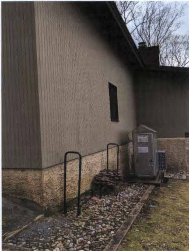
Existing north facing elevation of garage area to be renovated
