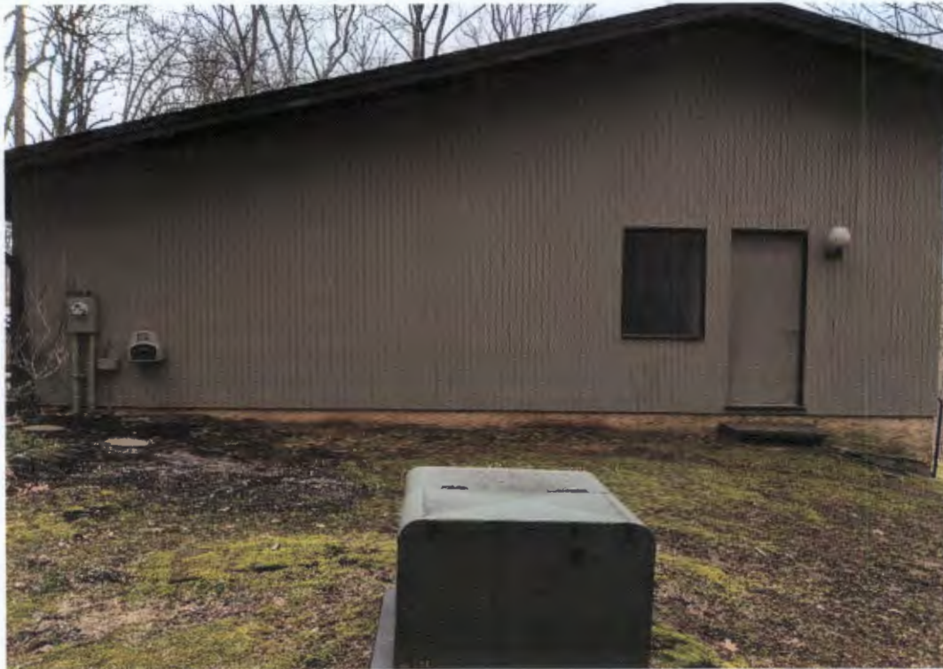
Existing east facing elevation of garage area to be renovated
