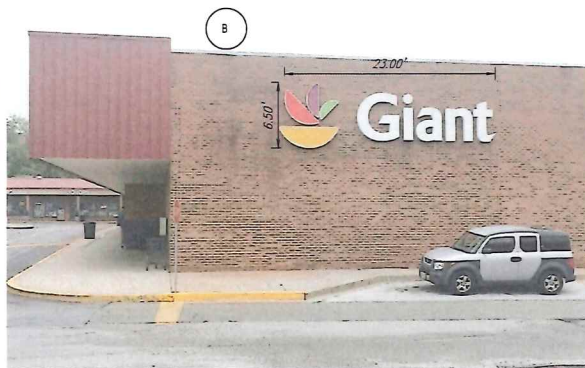
BUILDING 1 SOUTH ELEVATION (BLD1SB)
