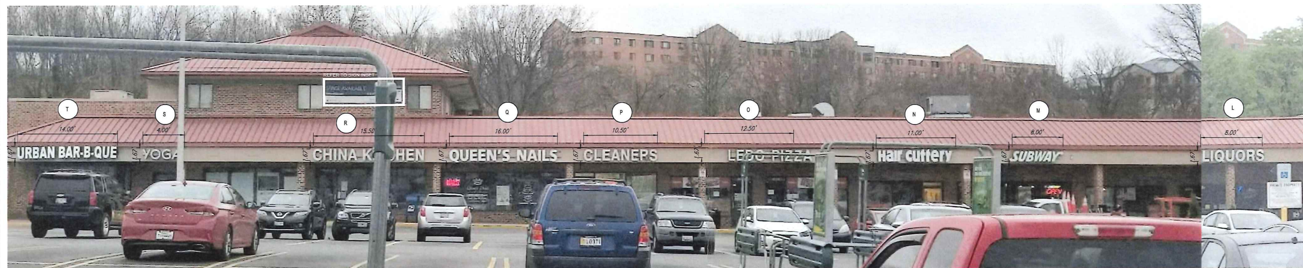
BUILDING 1 SOUTH ELEVATION (BLD1SA)
