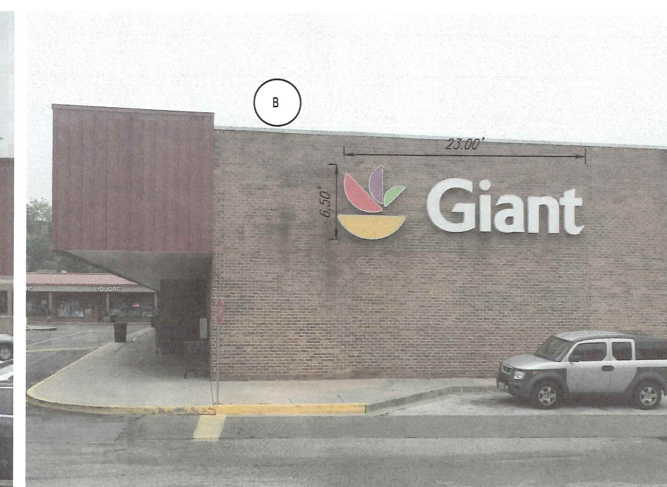
BUILDING 1 SOUTH ELEVATION (BLD1SB)
