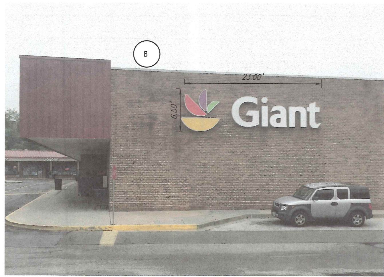
BUILDING 1 SOUTH ELEVATION BLD1SB
