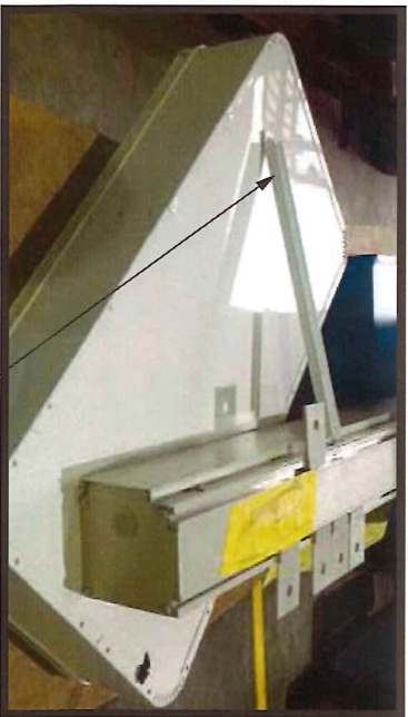
Added Bracing- bent channel attached to letters "R" & "T" - .063 painted white alum w/ machine screws *photo used is representational ONLY*
