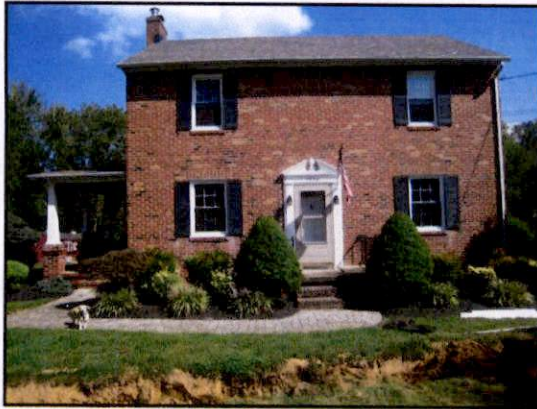
FRONT VIEW..GROUND IS DUG UP DUE TO NEW DRAIN FIELD CURRENTLY BEING INSTALLED (CHRIS MILAN) SUBURBAN CONTRACTOR
