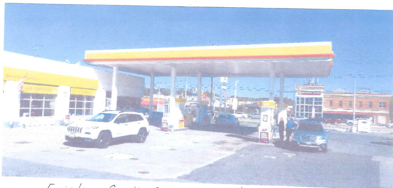
Existing South Canopy Elevation
