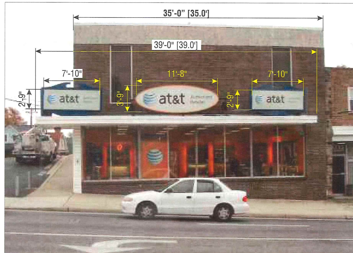
Three signs to be removed from this elevation
