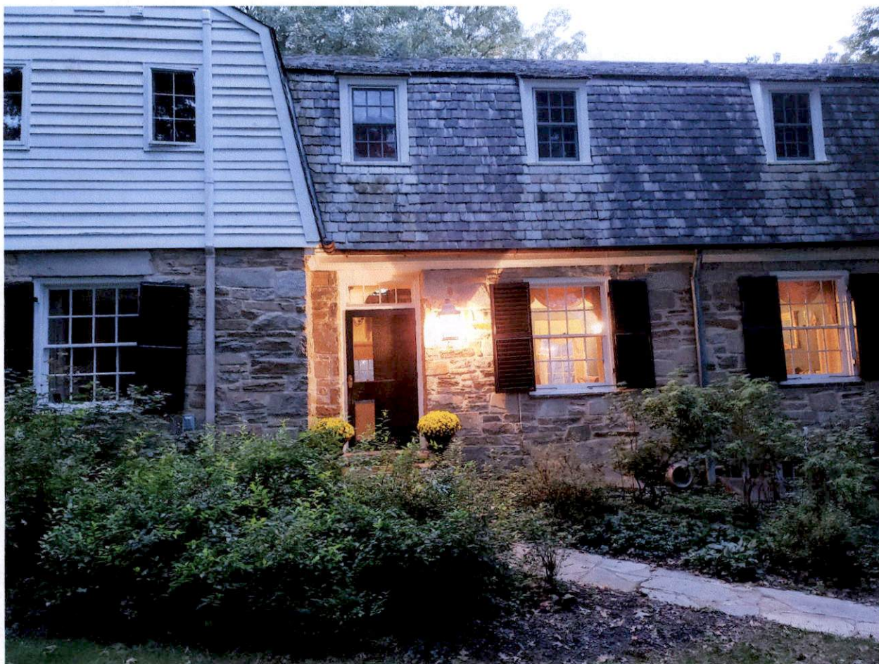
Front of house faces east, Seminary Road on north side of property.
