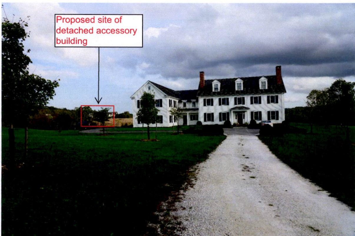
Photograph #2- From driveway towards front door of house
