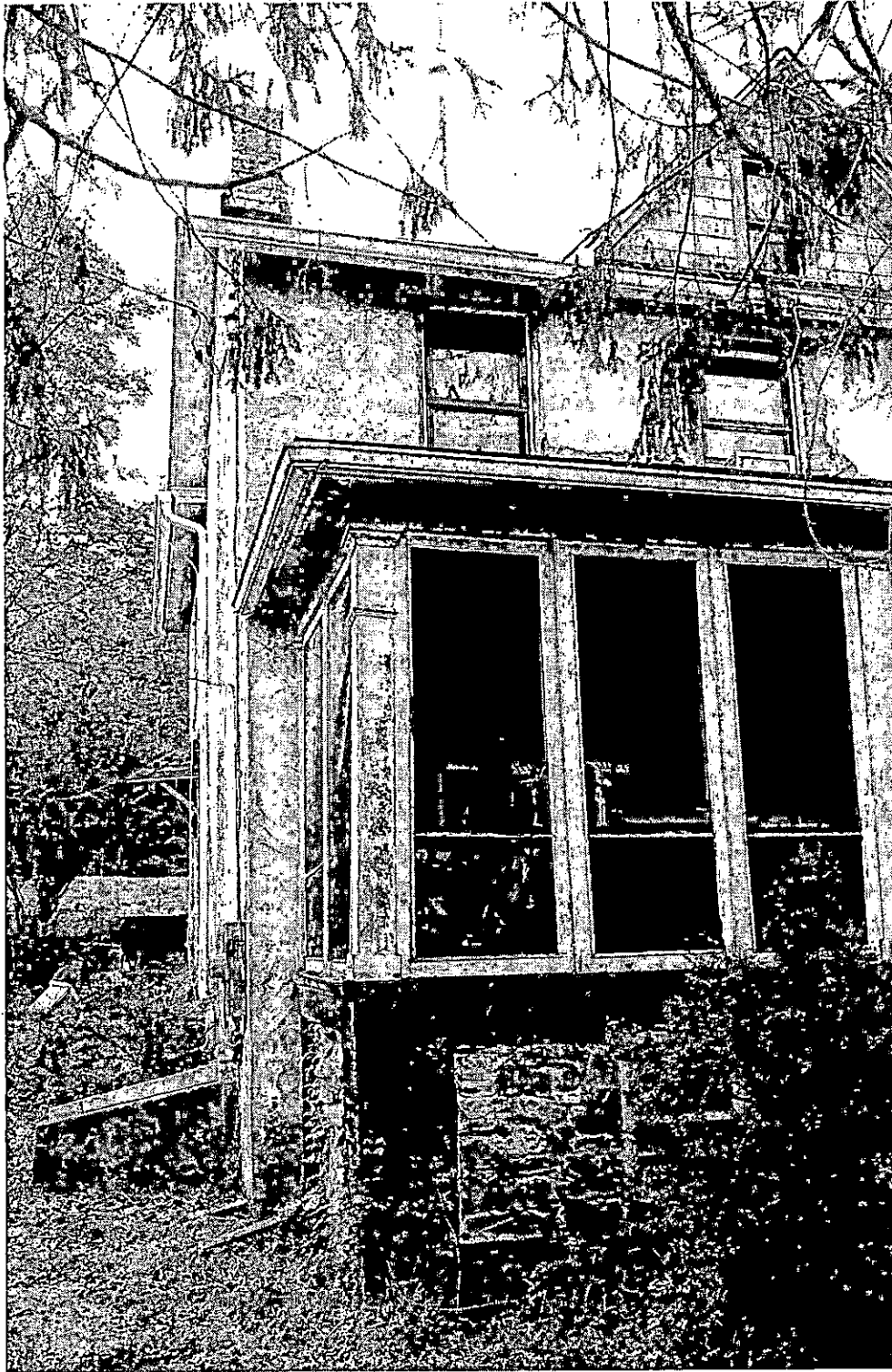
Front view, SW corner
