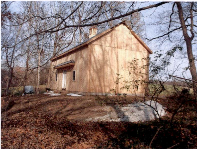
View looking North
