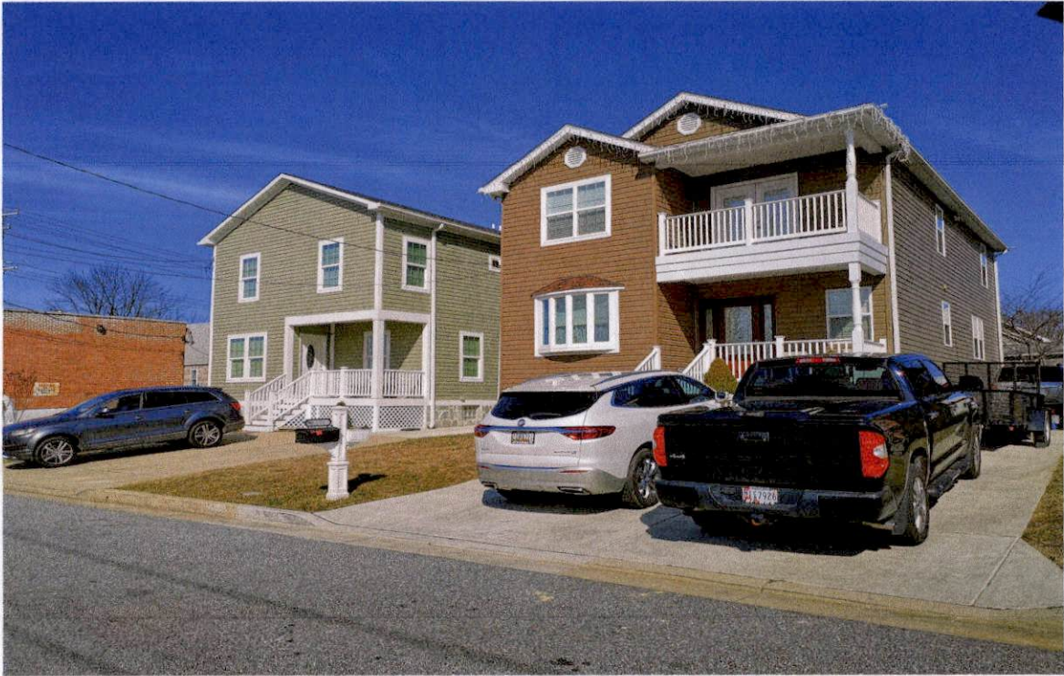
2802 Alabama Ave and 2804 Alabama Ave
