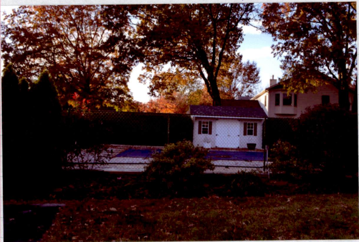
Facing west, showing elevation. Dwelling is to the right (out of the picture!)
