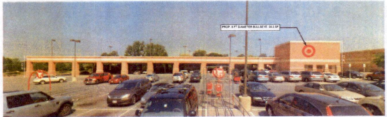
Parking Garage Southeast Elevation
