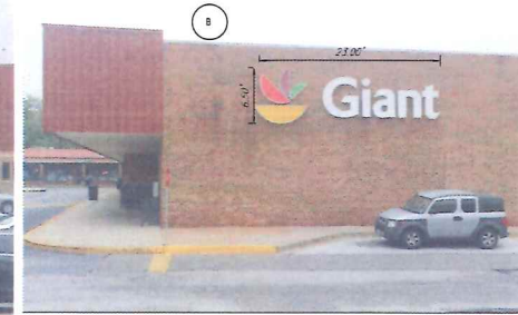
BUILDING 1 SOUTH ELEVATION BLD1SB
