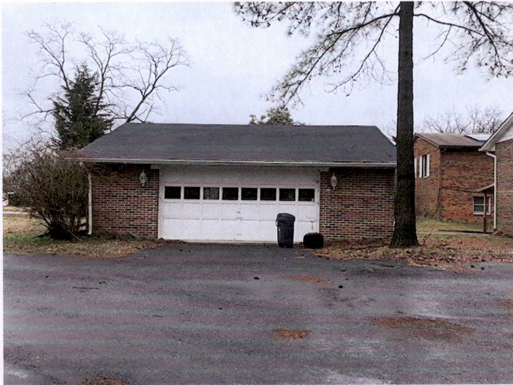
West side of garage
