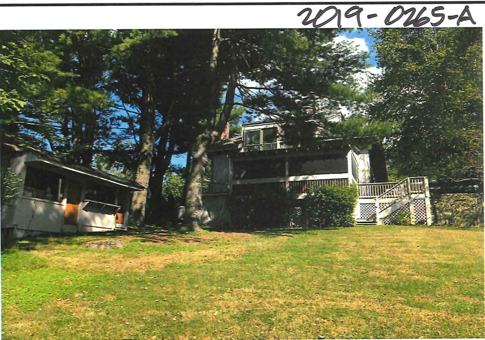
LOCATION OF ADDITION - HOUSE RIGHT SIDE W/ EXISTING OUTBUILDING TO REMAIN
