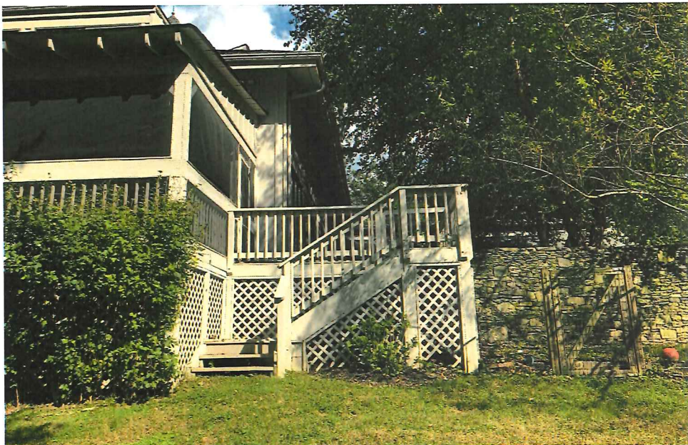
VIEW OF SOUTH WEST CORNER
