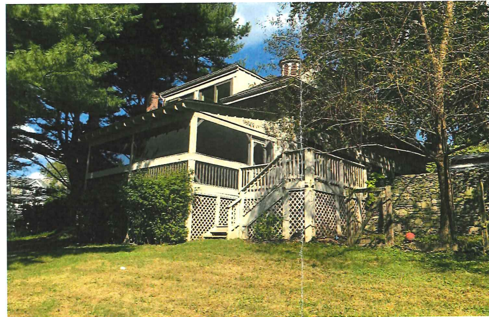
LOCATION OF ADDITION W/ (7350 BRIGHTSIDE) NEIGHBOR'S HOUSE BEYOND
