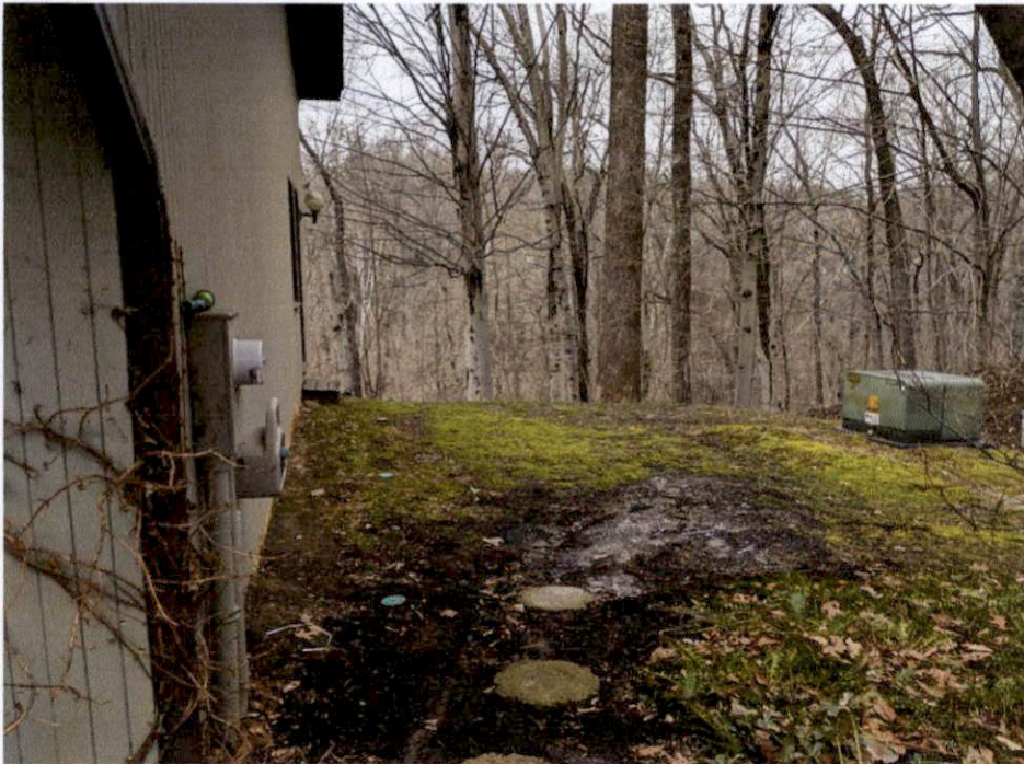
Looking north from existing garage. Property drops significantly in grade at back of structure towards Towson Run.
