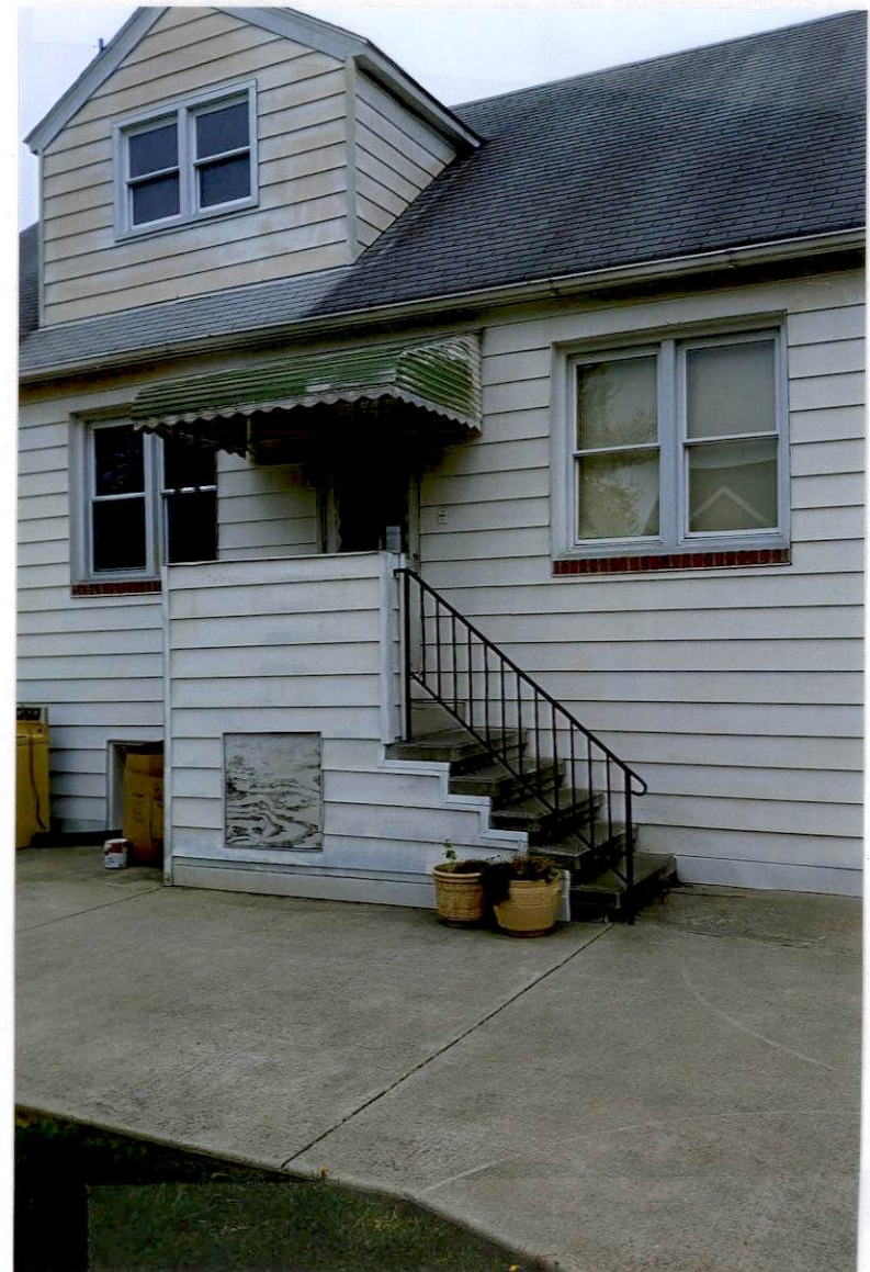
View of Side of House showing Entrance Door to 2nd Floor Unit 2019-0320-SPH
