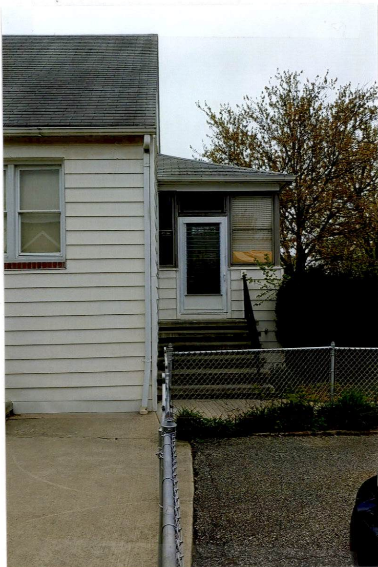
Front Door to Porch For 1st Floor Unit
