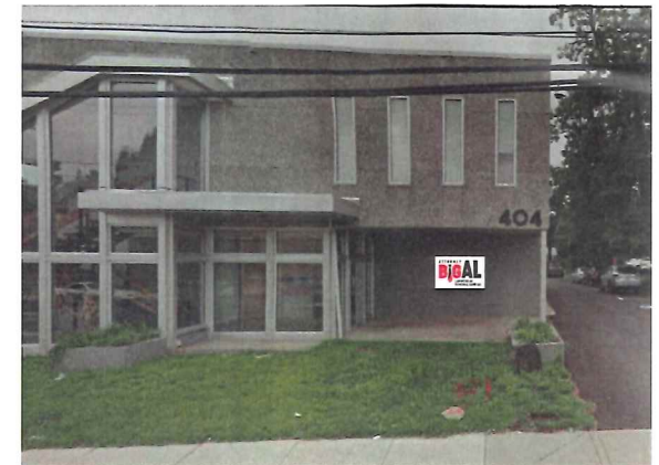
Building from Reisterstown Rd
