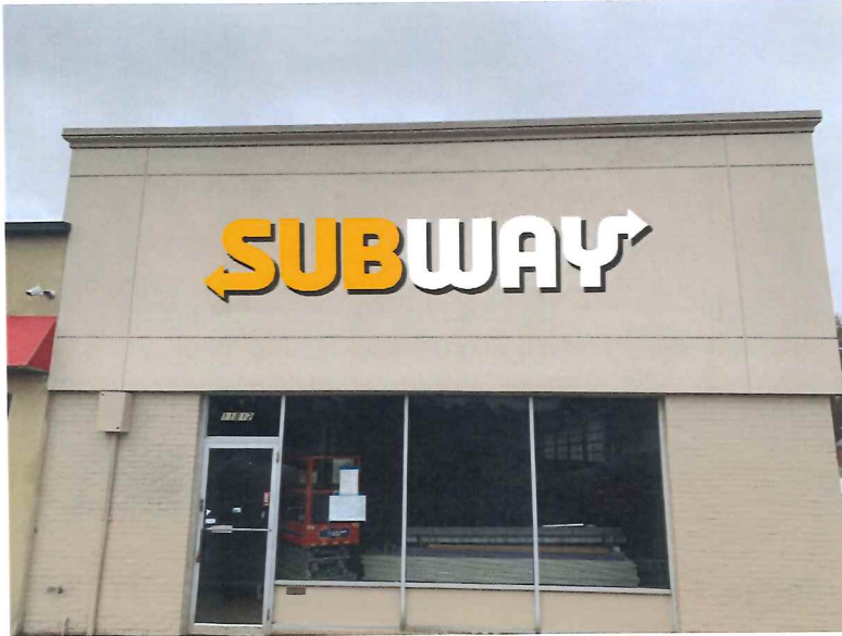
Signage at Front of Building
