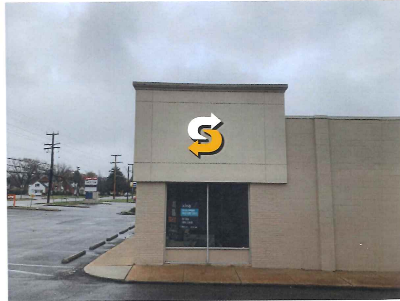
Signage at Side of Building
