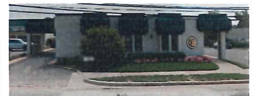
North facade - Street frontage 4 ft x 4 ft
