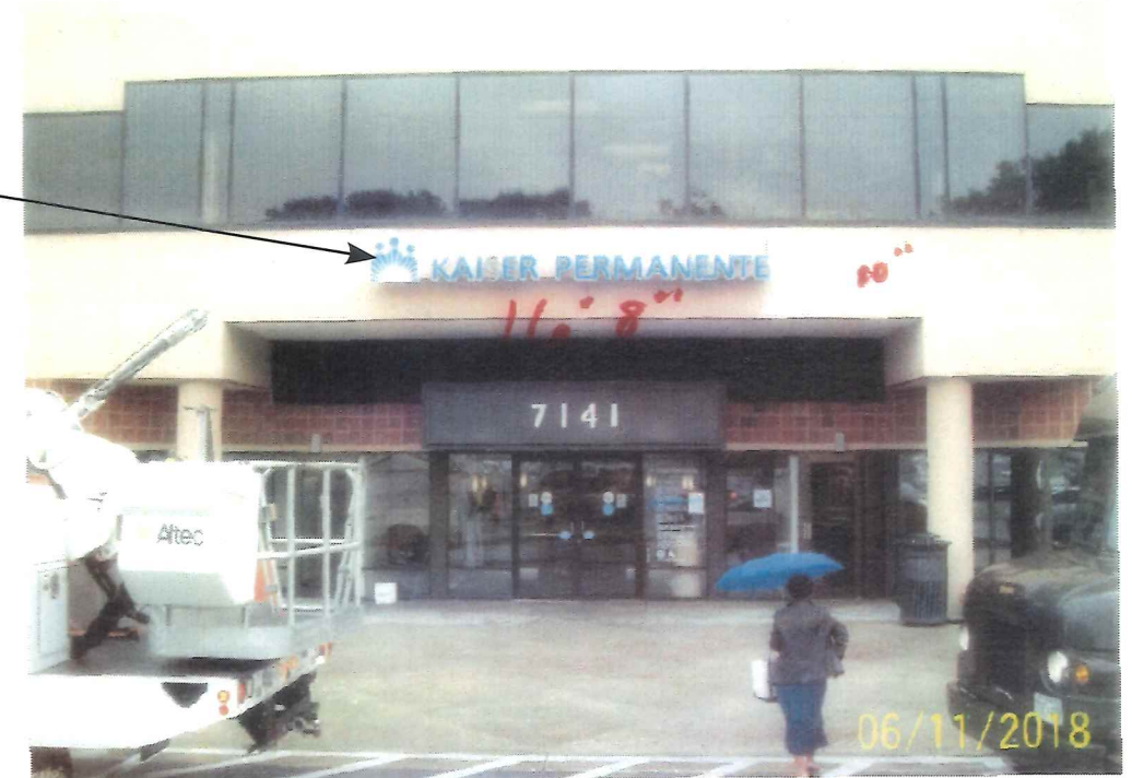
Photo showing existing sign
