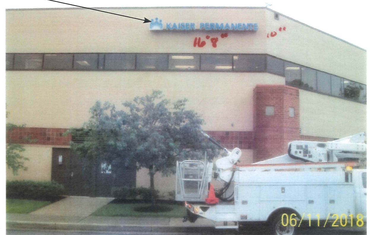
Photo showing existing sign
