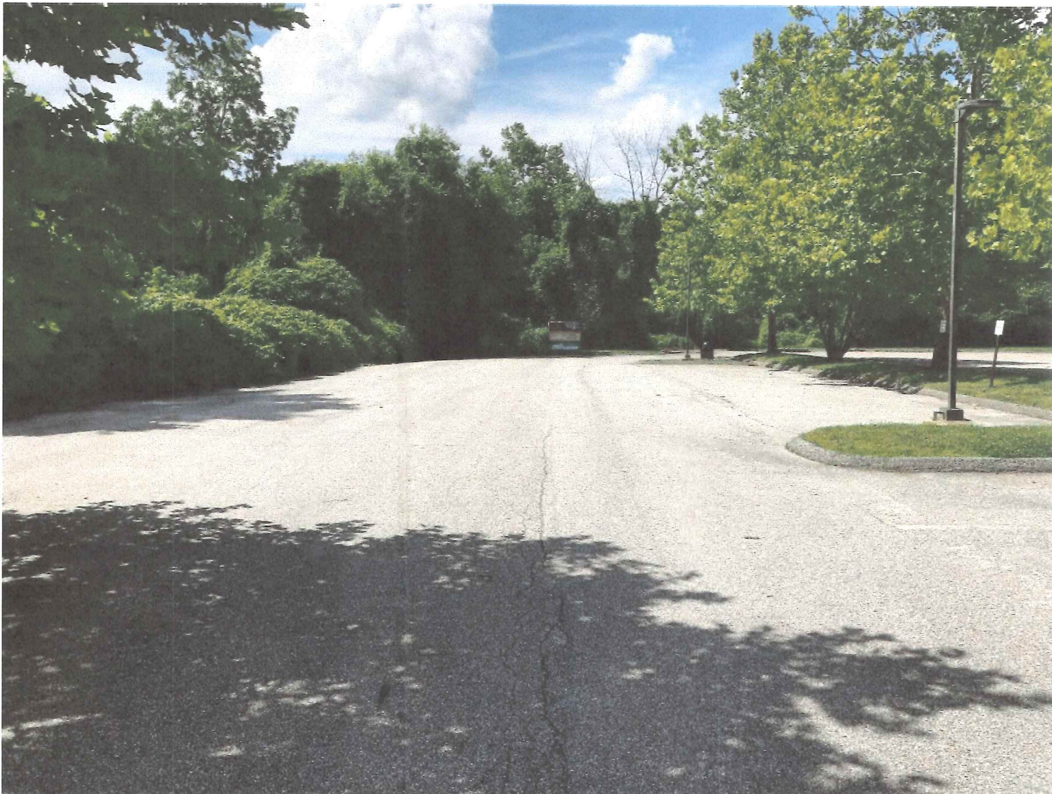
FUTURE VEHICLE STORAGE AREA
