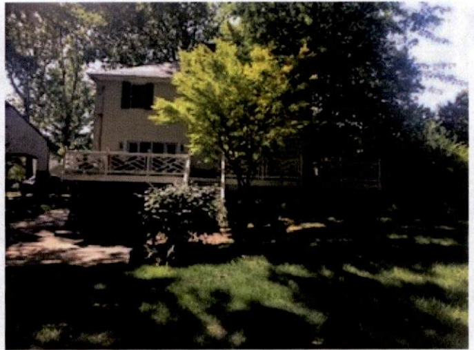
8 – Back Elevation – Facing East
