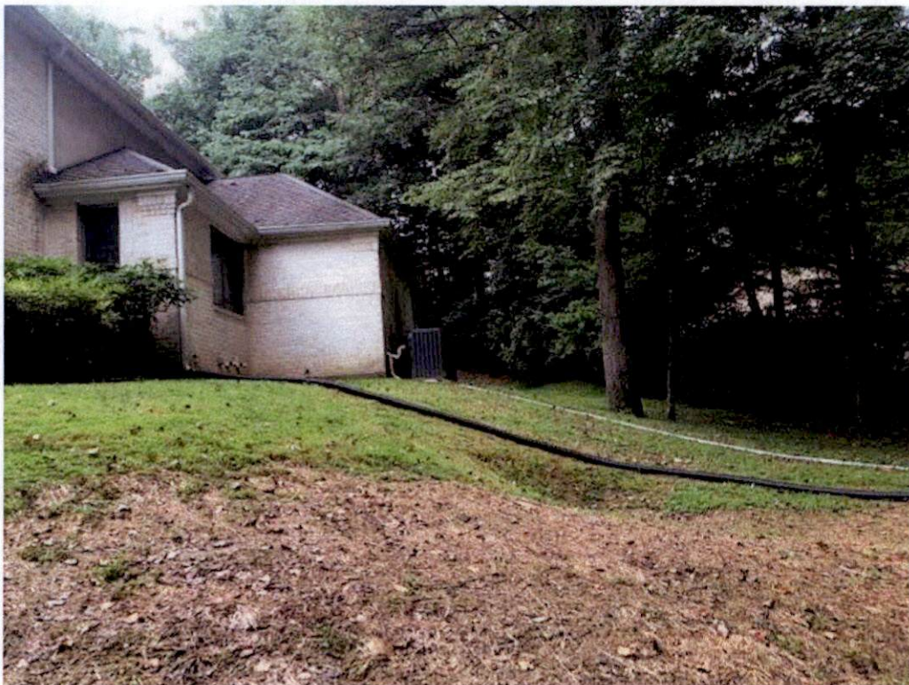
2. VIEW OF AREA TO GET ADDITION FROM FRONT OF HOUSE .
