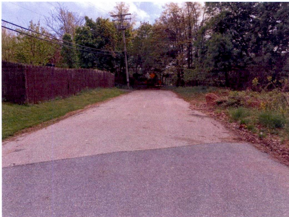
PHOTO#4: West Cherry Hill Road (Looking South from the Intersection)
