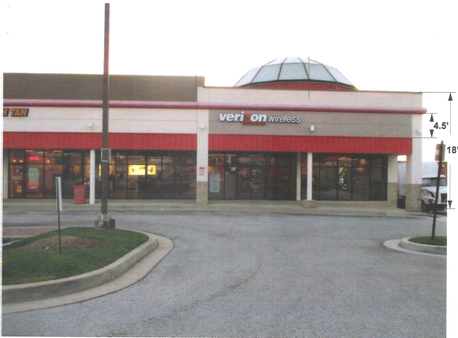
EXISTING SIGNAGE: EXISTING VERIZON SIGNAGE HEIGHT 16" V
