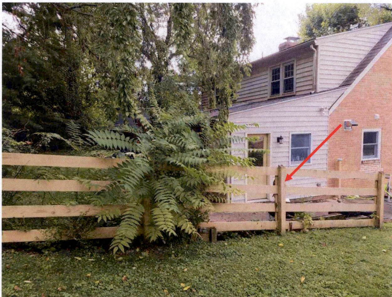
Back of 625 Debaugh from the west looking east, this is the site where the proposed garage will be, the west garage wall being exactly where the fence indicated by the red arrow is located.
