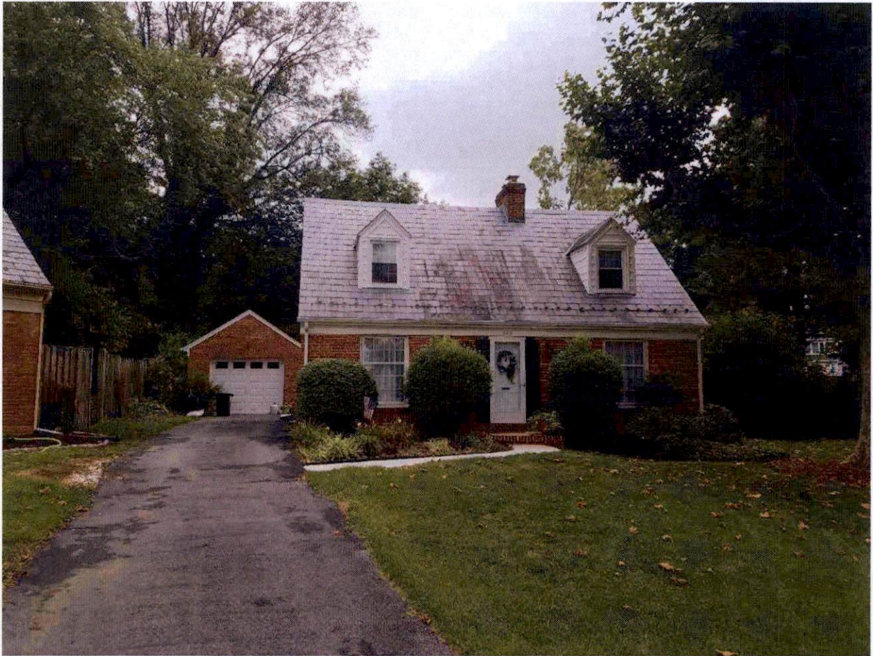
623 Debaugh. Proposed garage edition will have similar look to this house. Note that this garage appears to cross into the property line of 625 Debaugh property line. The edge of 625 Debaugh dwelling is just visible on the left of the image
