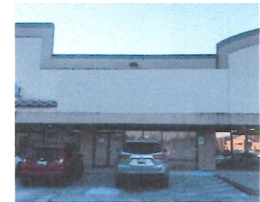
EXISTING STORE FRONT
