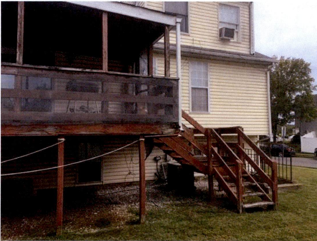
7107 OLIVER BEACH ROAD – EXISTING DECK
