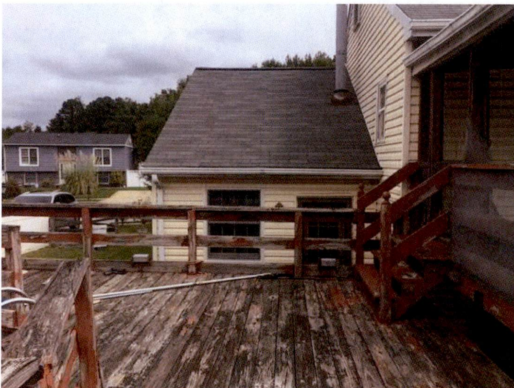
7107 OLIVER BEACH ROAD – EXISTING DECK
