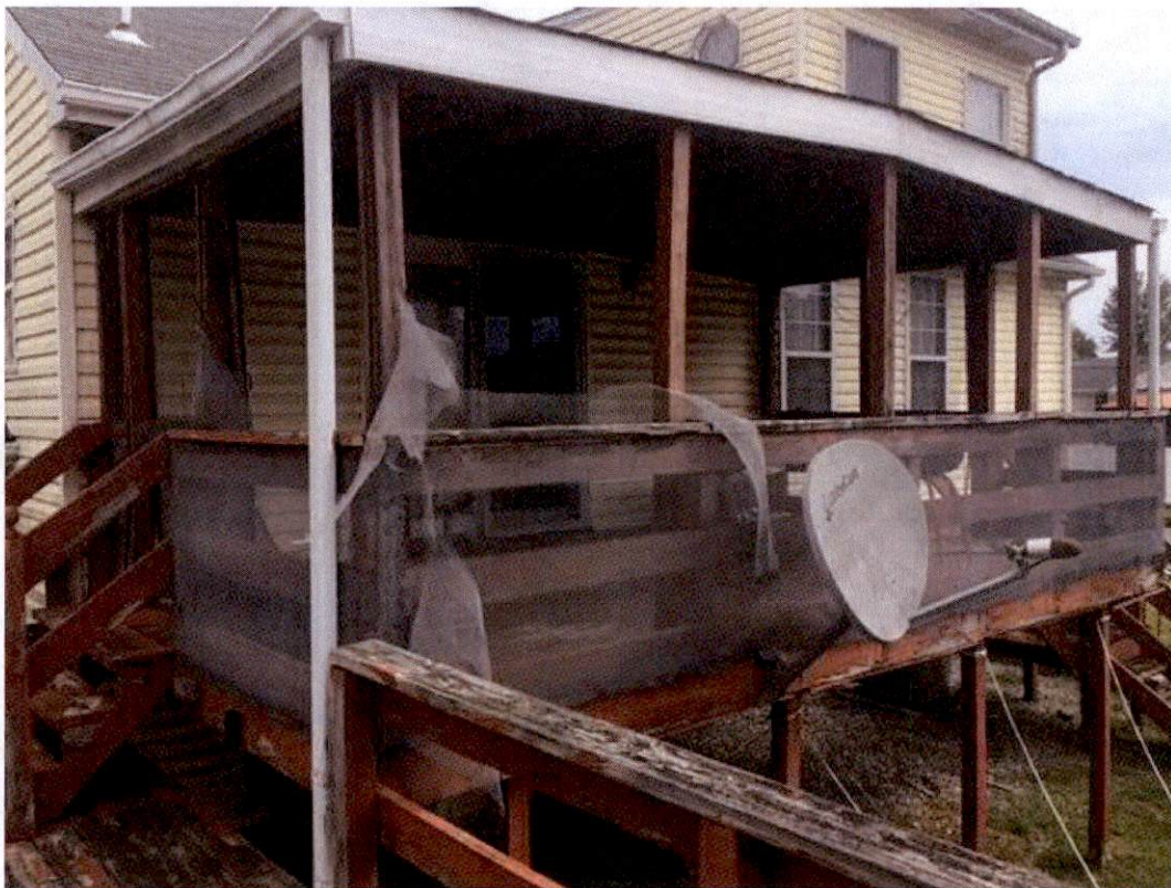
7107 OLIVER BEACH ROAD – EXISTING DECK
