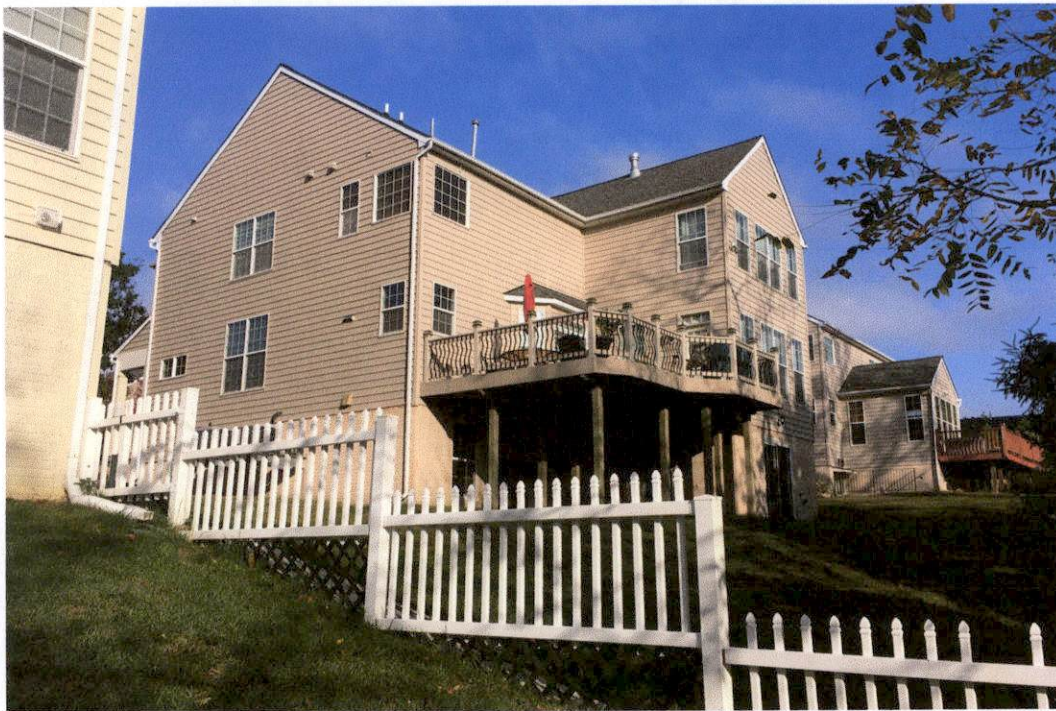
ANOTHER PICTURE SHOWING STEEPLY SLOPING LOT TOPOGRAPHY - TAKEN FROM INSIDE THE FENCE IN BACKYARD OF SUBJECT (2015 WILLOWCREST CIR)
