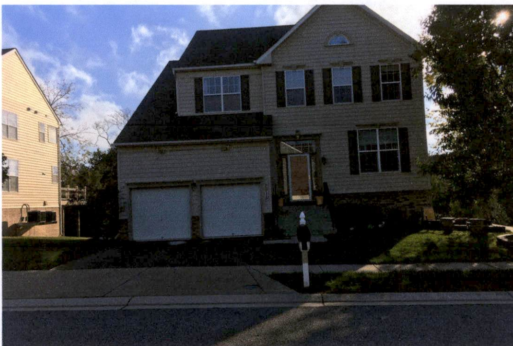
2015 WILLOWCREST CIRCLE (SUBJECT PROPERTY) - PICTURE OF THE PROPERTY FRONT - TAKEN FACING EAST
