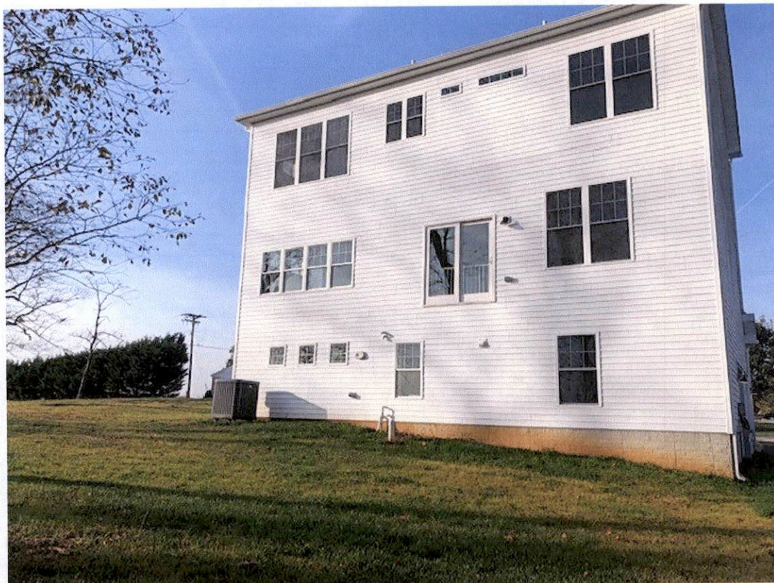
Rear of house
