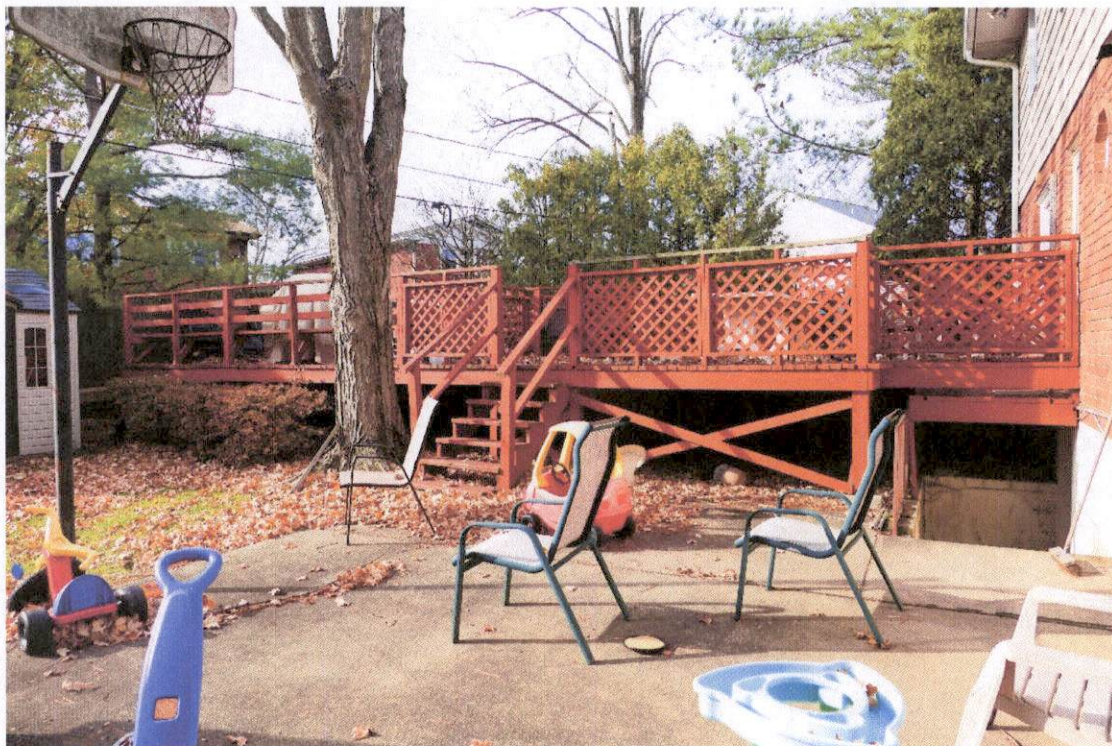
House deck and shed
