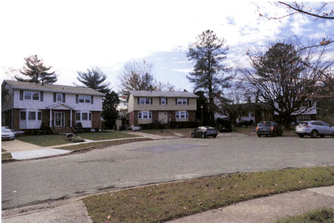
Left to right: 2703, 2705 and 2707 Copperfield Court
