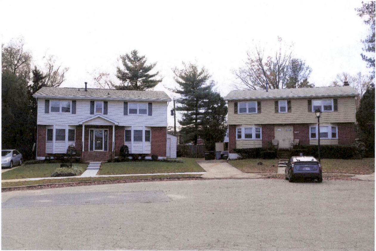
2703 and 2705 Copperfield Court
