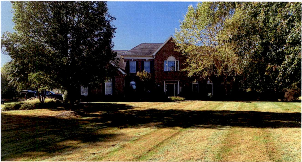
1 Front House from Looking South from Belfair Lane
