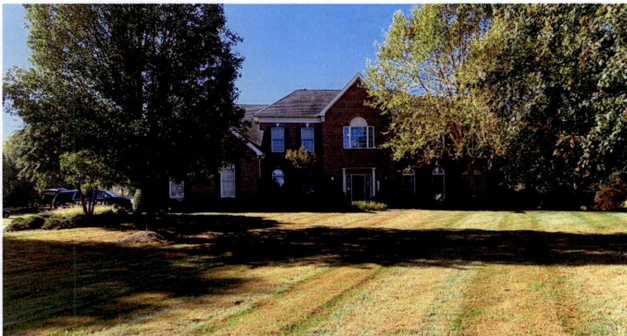
1 Front House from Looking South from Belfair Lane
