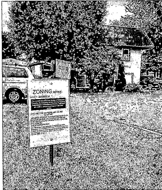
Background Photo 1 st Sign @ 9707 Pulaski Highway ~ 5/28/2020
