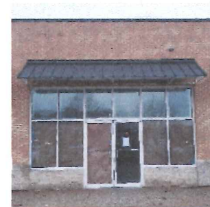
EXISTING STORE FRONT
