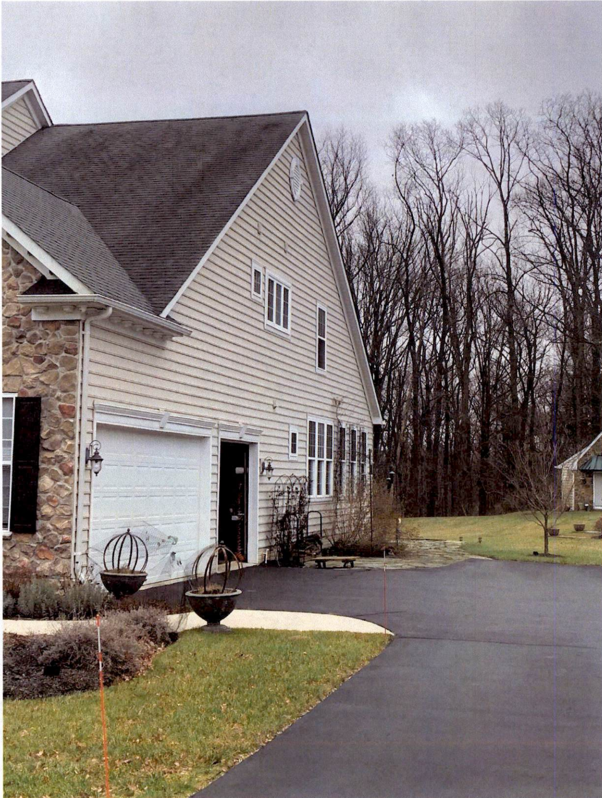
Garage Side Elevation – Right Side (close-up) (Proposed extension of mudroom this side)
