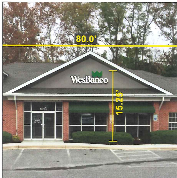
Face-lit channel letters on raceway
