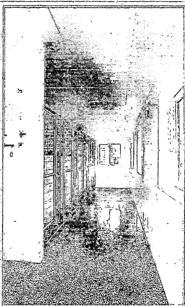
Interior View Of 10x28 5-Run kennel with 3' overhang with 10' Add-on runs. Showing welded wire panels and exhaust fan.
