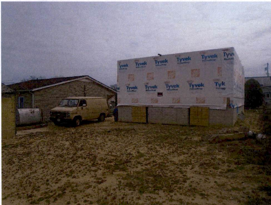
March 18, 2020 – Rear View of Partially Constructed House
