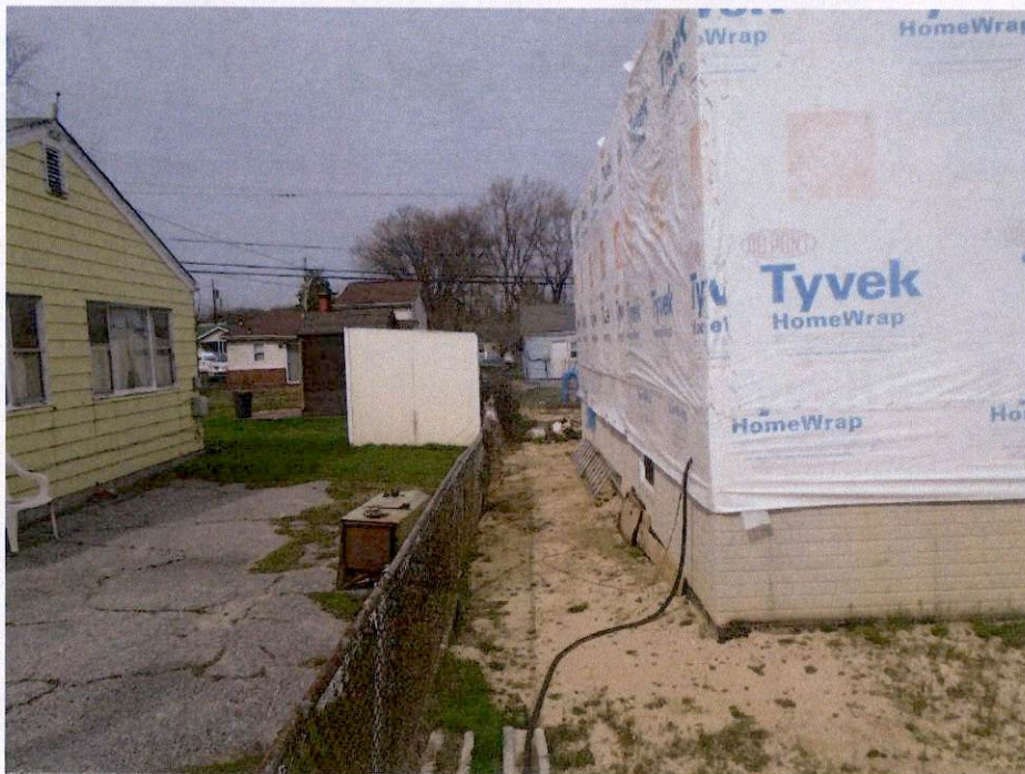
March 18, 2020 – Left Side of Partially Constructed House
