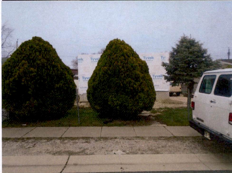
March 18, 2020 – Front View of Partially Constructed House
