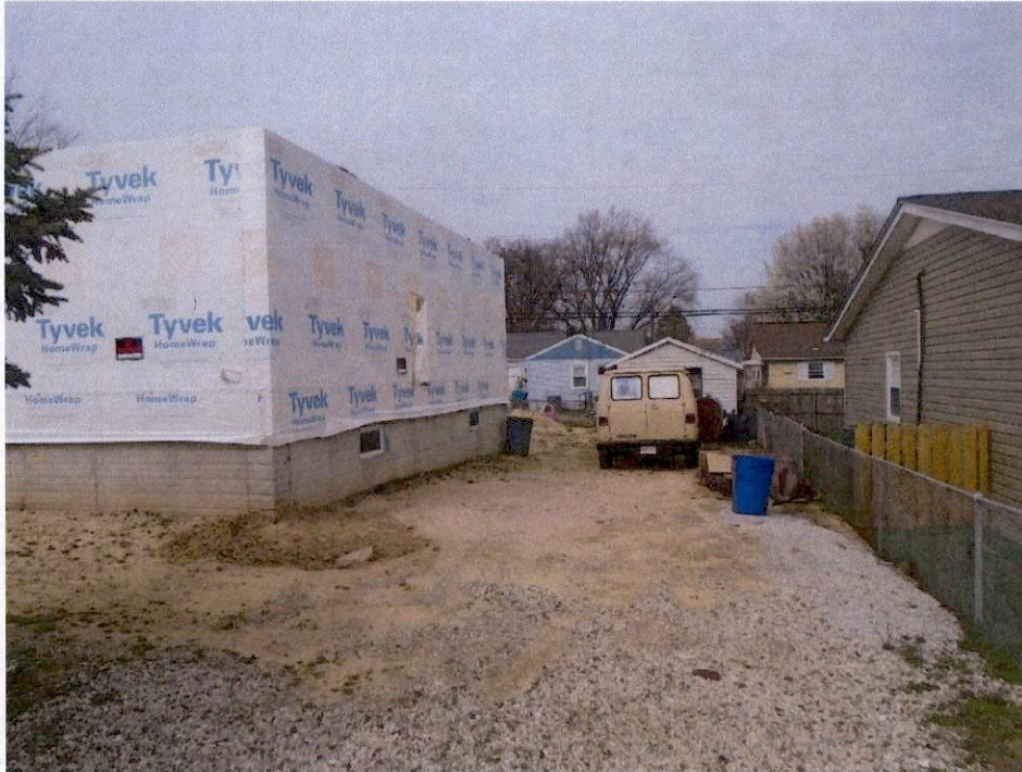
March 18, 2020 – Right Side of Partially Constructed House
