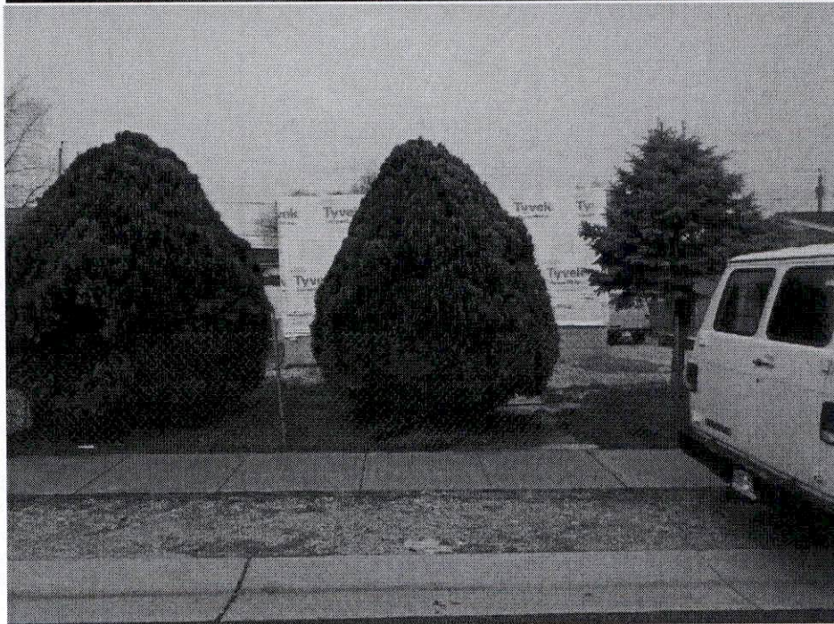
March 18, 2020 – Front View of Partially Constructed House
