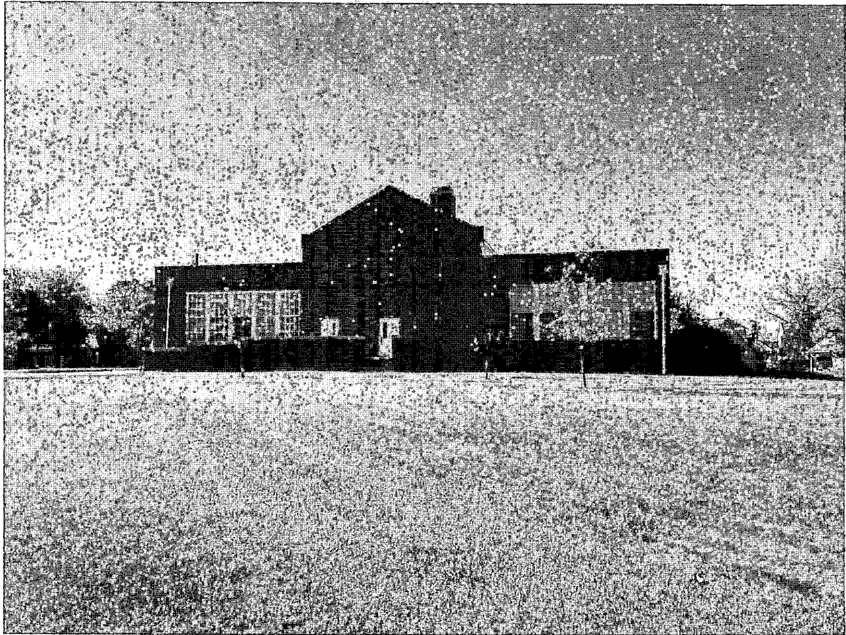
VIEW OF EXISTING BUILDING - REAR
