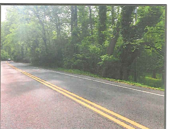
13 - VIEW TOWARD NORTHWEST @ OLD COURT ROAD
