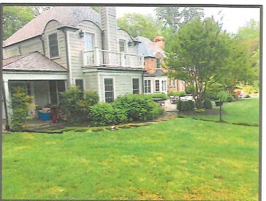
8 - VIEW FROM SW BACK TOWARD HOUSE
