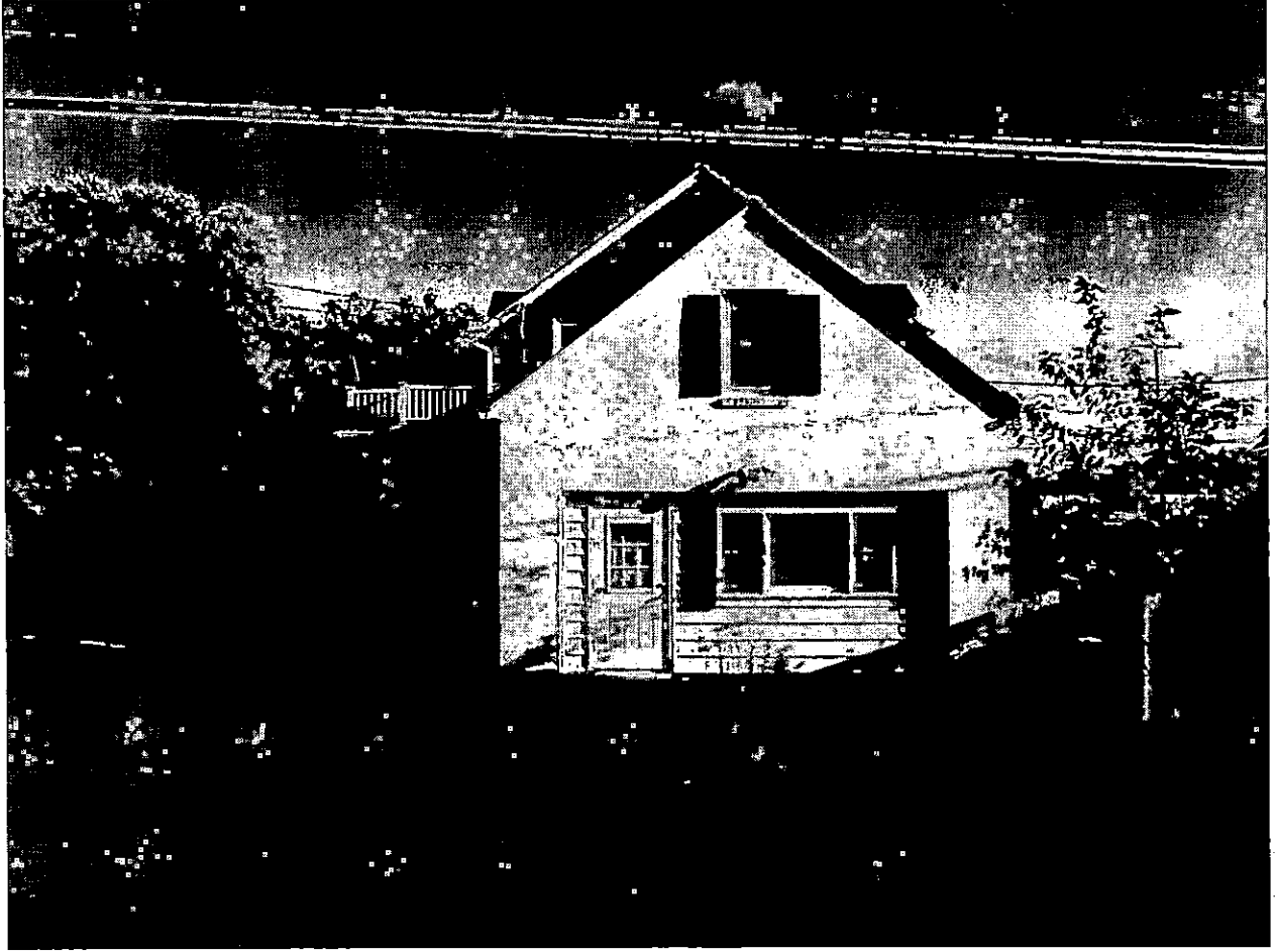
October 8 th , 2020-Photograph from opposite side of Virginia Avenue facing toward northwest side of 11723 Reisterstown Road. Photo taken facing southeast, toward building. Virginia Avenue is in the foreground and Reisterstown Road is to the right of the photo.
