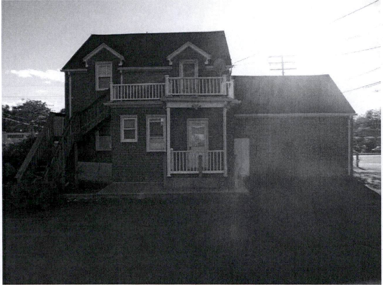
October 8 th , 2020-Photograph from rear parking lot of 11723 Reisterstown Road, facing southwest toward building and Reisterstown Road. Virginia Avenue is to right of photo.
